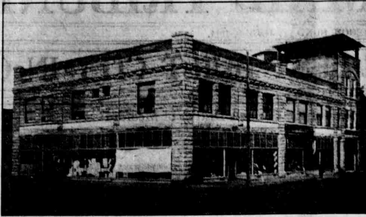
St. Marks block, completed within the past year by the St. Marks Episcopal church.
