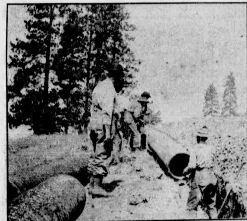
LAYING 18-INCH MAIN THROUGH MOUNTAINS.
