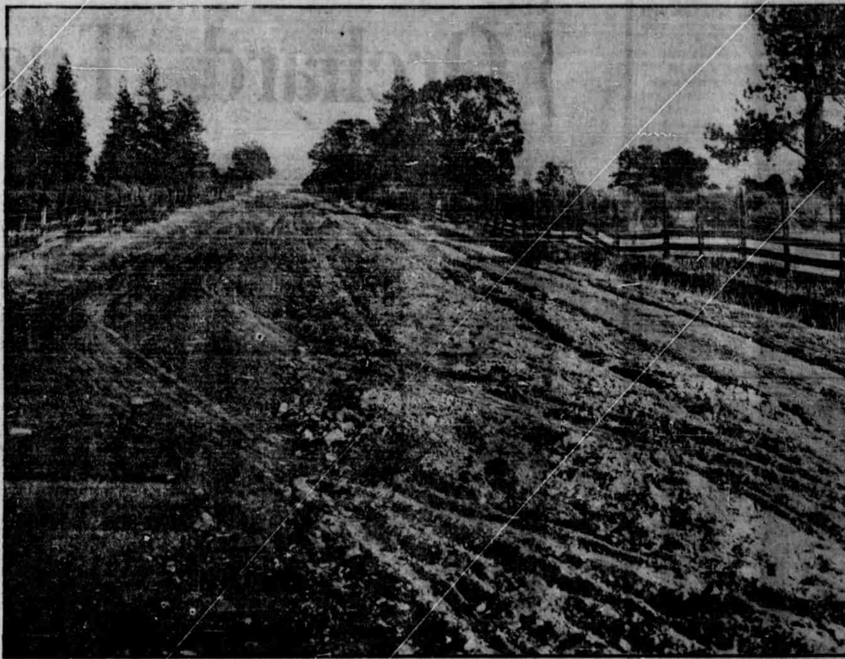
Photograph of "Little Sticky" lane, a county road, a mile in length, connecting the Eagle Point and Central Point roads. It illustrates road building as practiced by County Commissioner Patterson. Built over a year ago, by dumping gravel in the center of the road, it has never been rolled or surfaced and is almost impassable. Vehicles are compelled to drive in the ditch on either side, until mud forces them over the gravel piles. There are many such stretches of "completed" roads in Jackson county.
