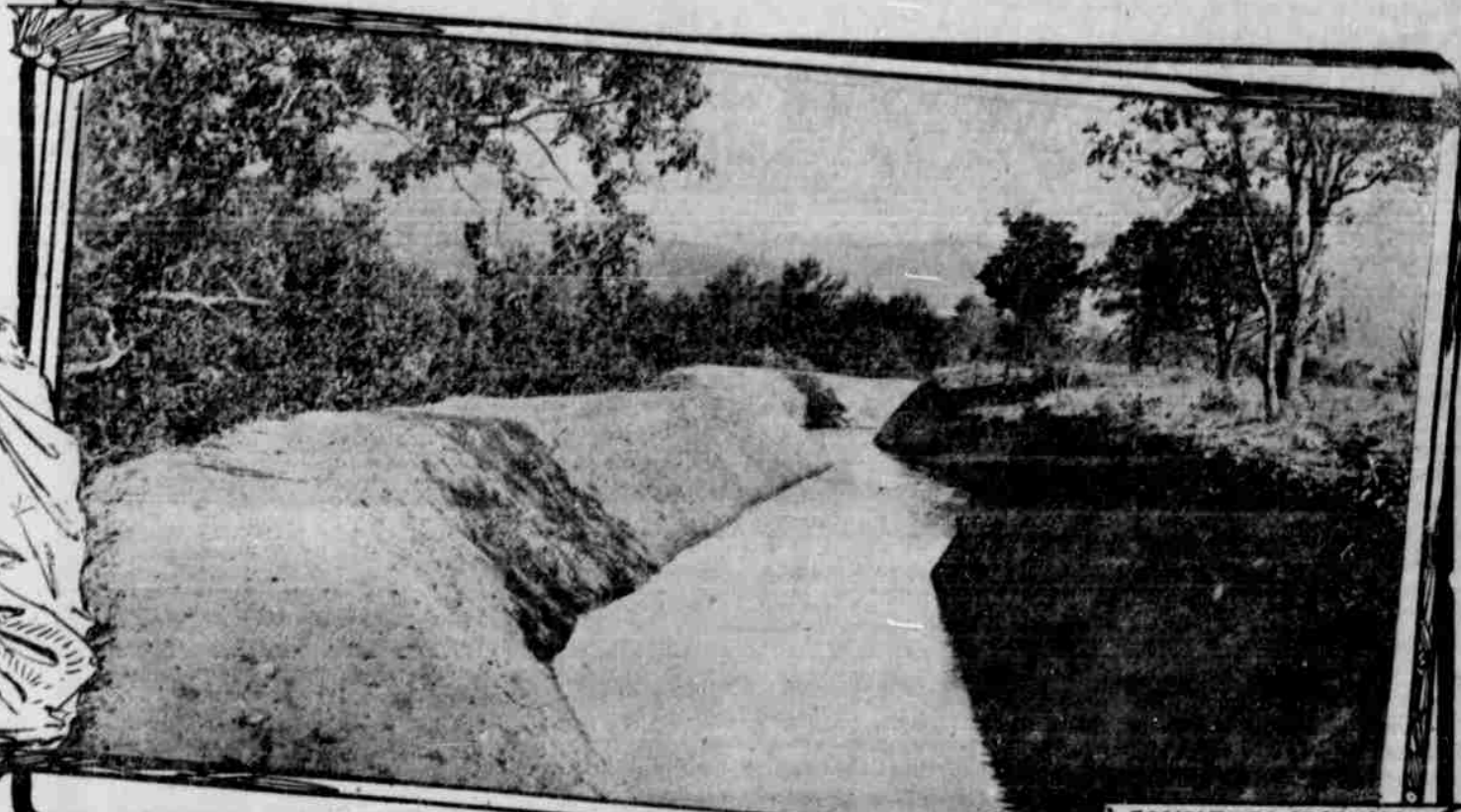
COMPLETED SECTION OF ROGUE RIVER VALLEY CANAL CO'S IRRIGATION CANAL TWELVE MILES EAST OF MEDFORD
