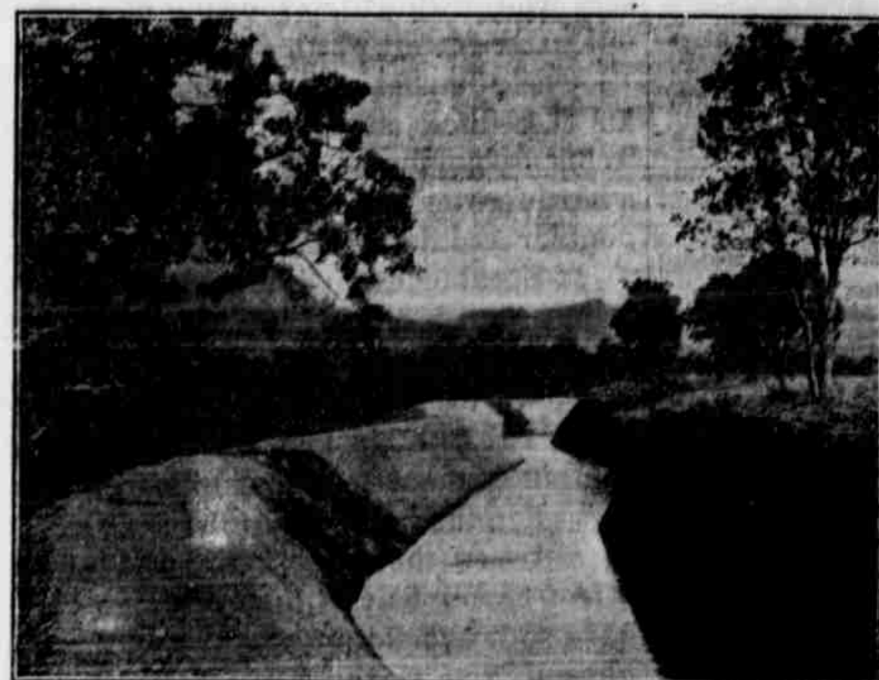
Completed Section of New Canal
