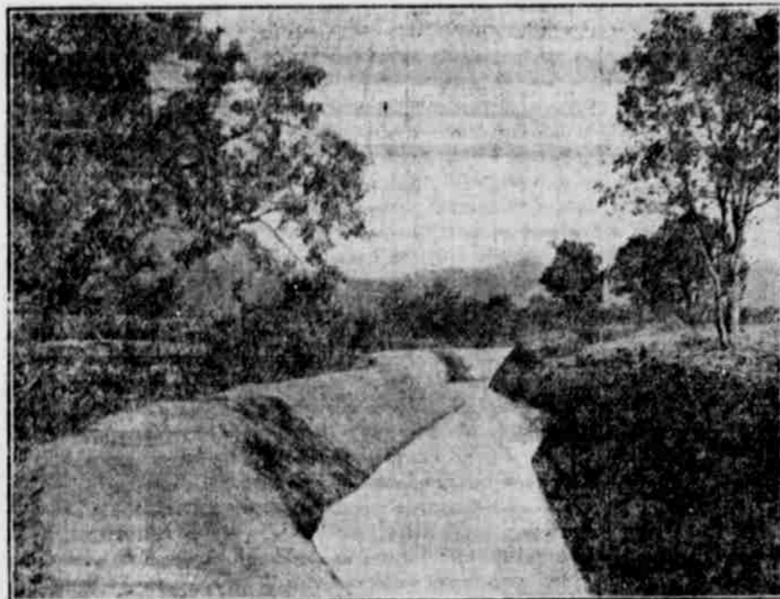
Completed Section of New Canal
