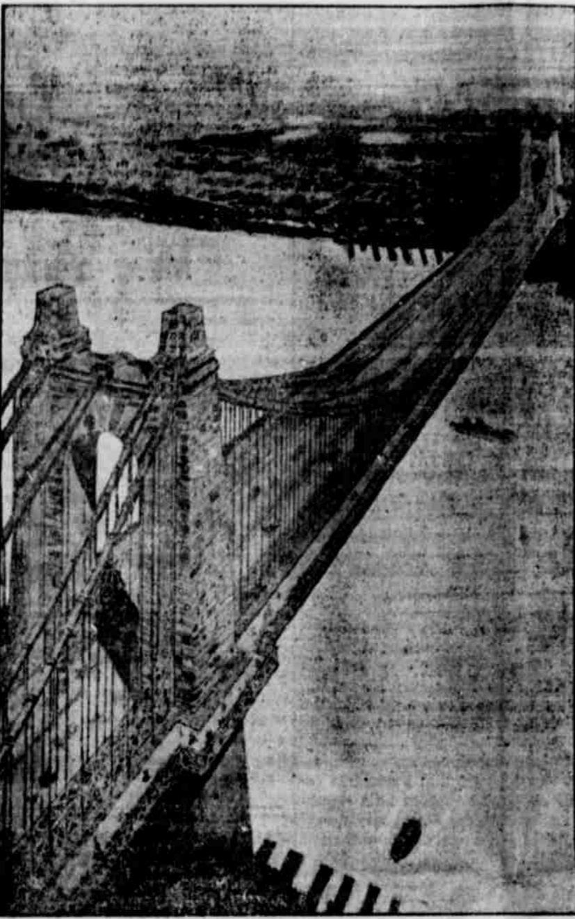
New York and New Jersey will be connected by one of the greatest bridges in the world. After long years of discussion work has at last been started on a $10,000,000 bridge that will reach from near Fort Lee, N. J. to Manhattan Island at One Hundred and Seventy-ninth street. The new bridge will dwarf Brooklyn bridge in size.
