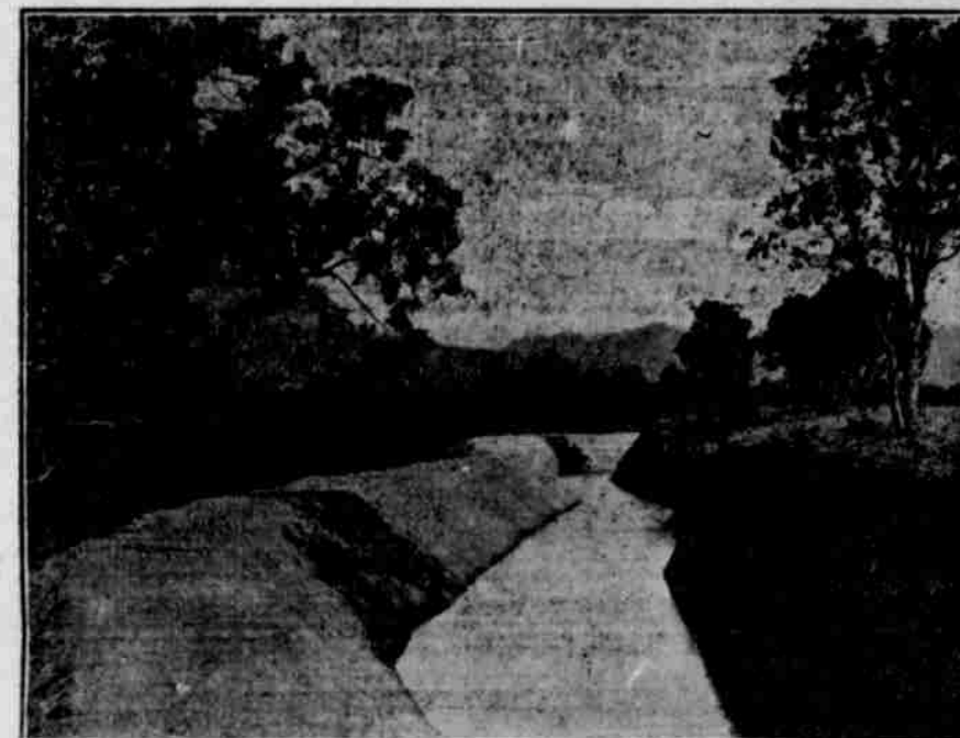
Completed Section of New Canal.
