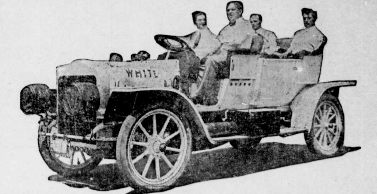
THE WHITE STEAMER WHICH MADE A SUCCESSFUL PUBLIC DEMONSTRATION OF KEROSENE AS FUEL ON THE RECENT 265-MILE GLIDDEN TOUR.
