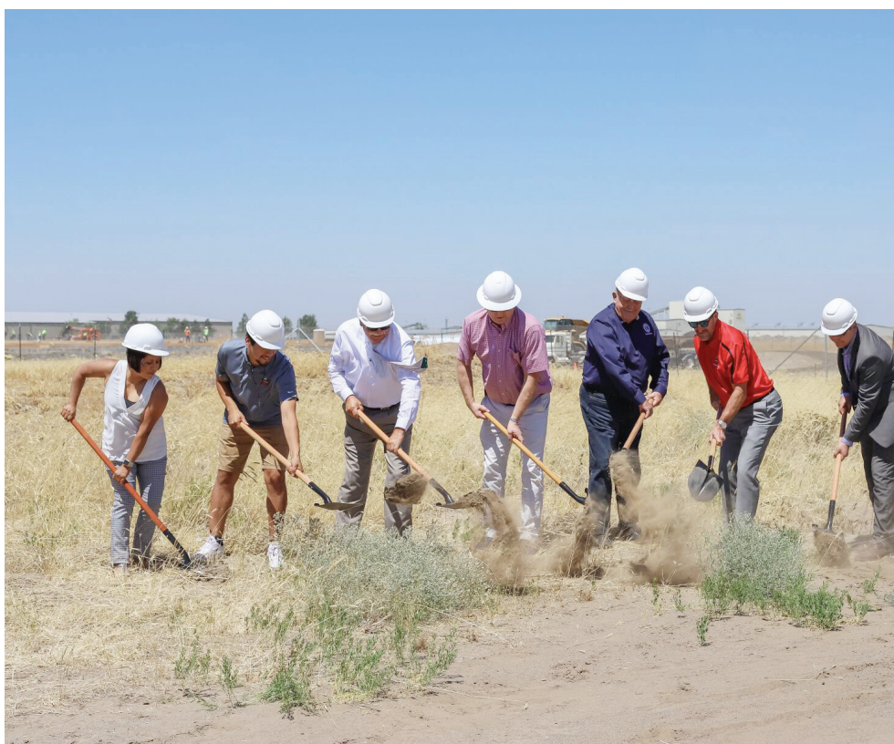
City of Hermiston/Contributed Photo, File From left, Hermiston City Councilors Maria Duron and Roy Barron, Umatilla County Commissioners Dan Dorran, John Shafer and George Murdock, Hermiston Mayor Dave Drotzmann and Assistant City Manager Mark Morgan break ground on the South Hermiston Industrial Park on July 7, 2021. The expansion now is complete with infrastructure ready for businesses to move in.
