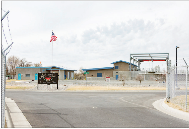
The Hermiston City Council voted to refinance loans taken out to pay for the city of Hermiston's wastewater treatment plant.
