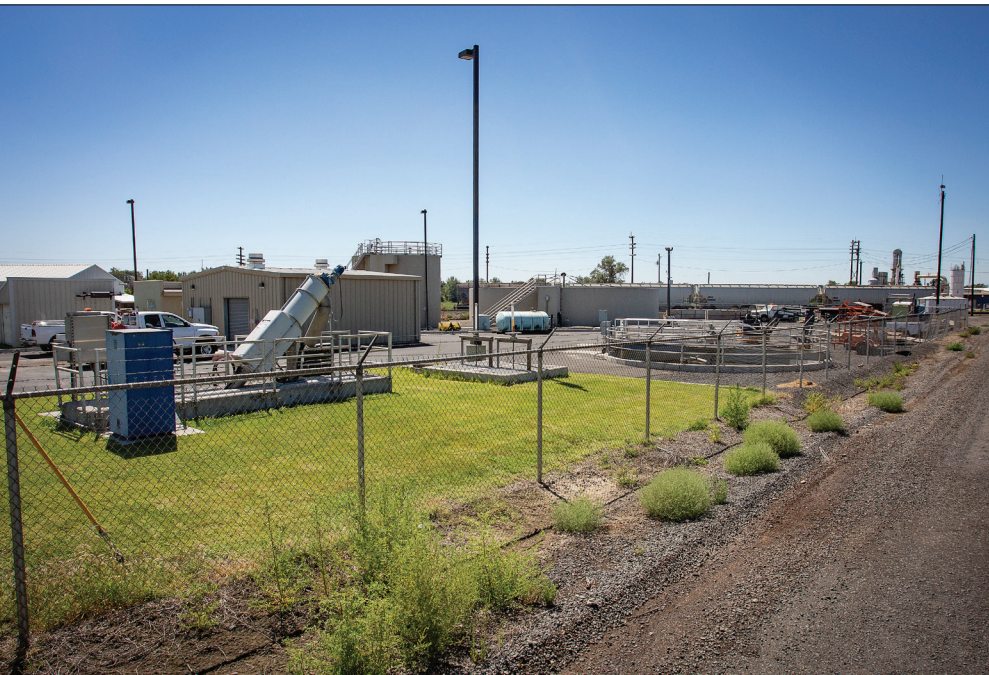
Staff photo by Ben Lonergan The city of Echo recently received $1.7 million in funding for upgrades to its wastewater infrastructure. One of the primary upgrades will be the installation of a pipeline to link the Echo system to the city of Stanfield’s wastewater treatment facility.
