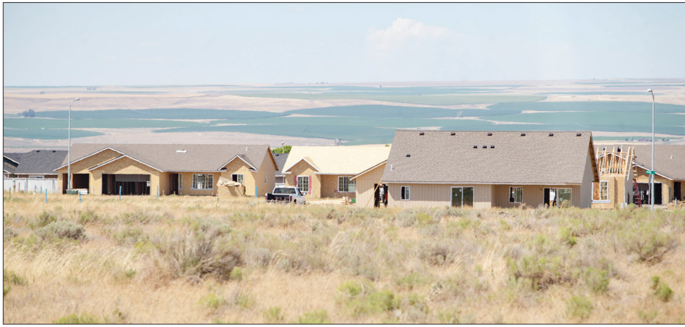
Homes sit in differing states of construction at a development along Powerline Road in Umatilla on Monday, July 6, 2020.
