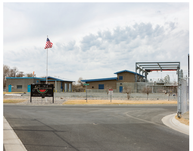
The city of Hermiston's wastewater treatment plant, constructed in 2014, was one of several capital projects that resulted in the need to raise water rates.
