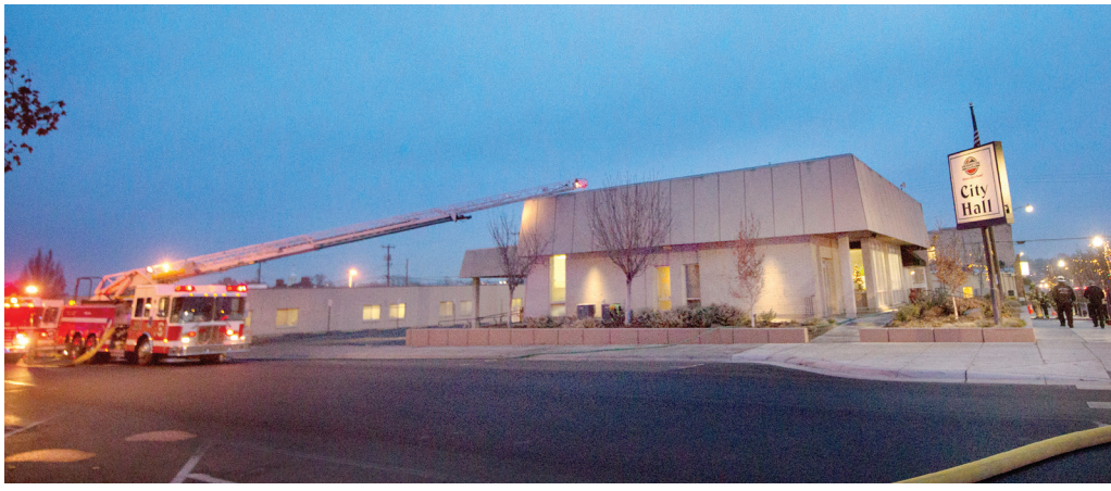
A fire engine sits at the ready Tuesday evening as firefighters check out the smoking interior of the Hermiston City Hall.
