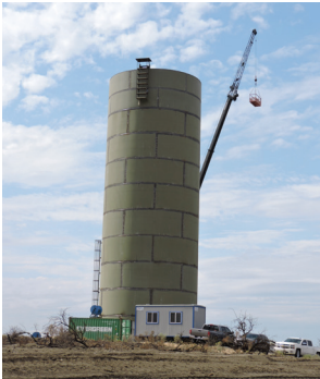
Staff photo by Jade McDowell A new water tower on the corner of Northeast 10th Street and Punkin Center Road in Hermiston is in the final stages of construction.
