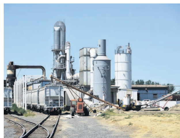
The 3D Idapro Solutions plant in Stanfield is receiving nearly a citation a day for odor complaints from residents of the town. HH FILE PHOTO
