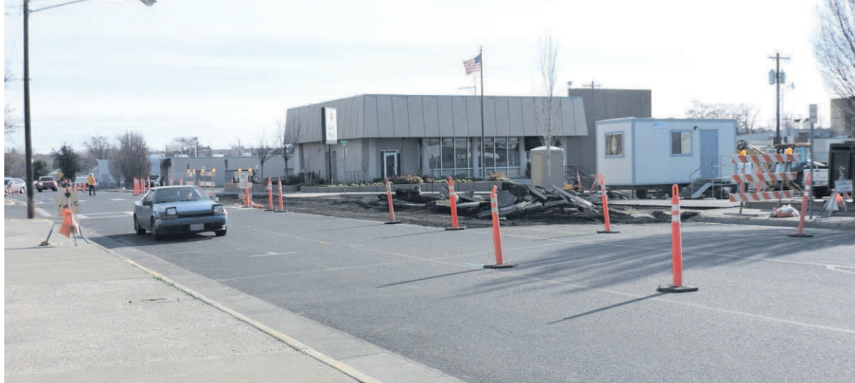
A car passes through the cones re-routing traffic near city hall.
