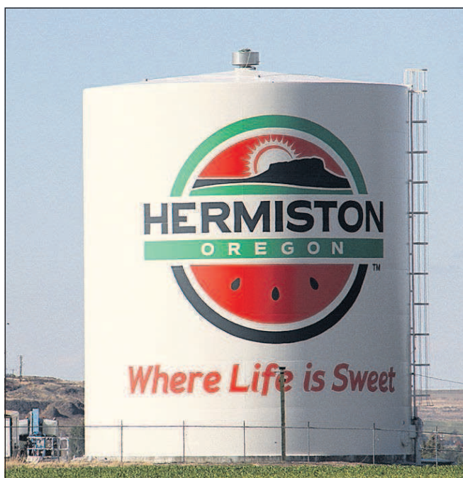
The Hermiston water tower got a fresh coat of paint and new logo in October, replacing the former "You Can GROW Here" slogan.
