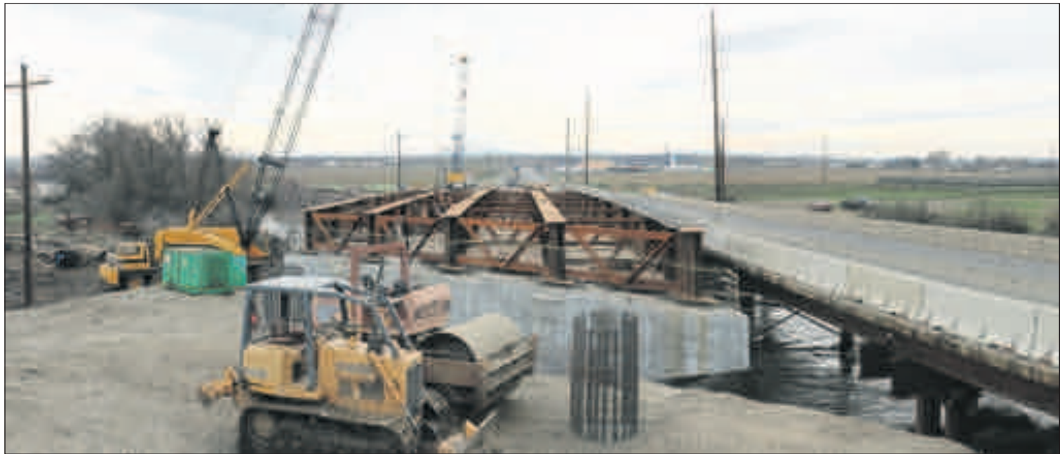
Construction of the Hinkle Bridge south of Hermiston.
