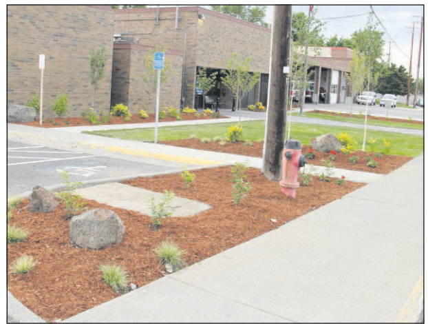
SEAN HART PHOTO Hermiston Parks and Recreation Director Larry Fetter designed the new landscaping in front of the Hermiston police and fire stations to comply with a proposed landscaping ordinance for new developments in the city.
