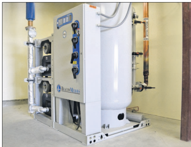
The surgical expansion at Good Shepherd Medical Center features high-tech equipment, including this vacuum control unit that senses when a person comes near the device.
