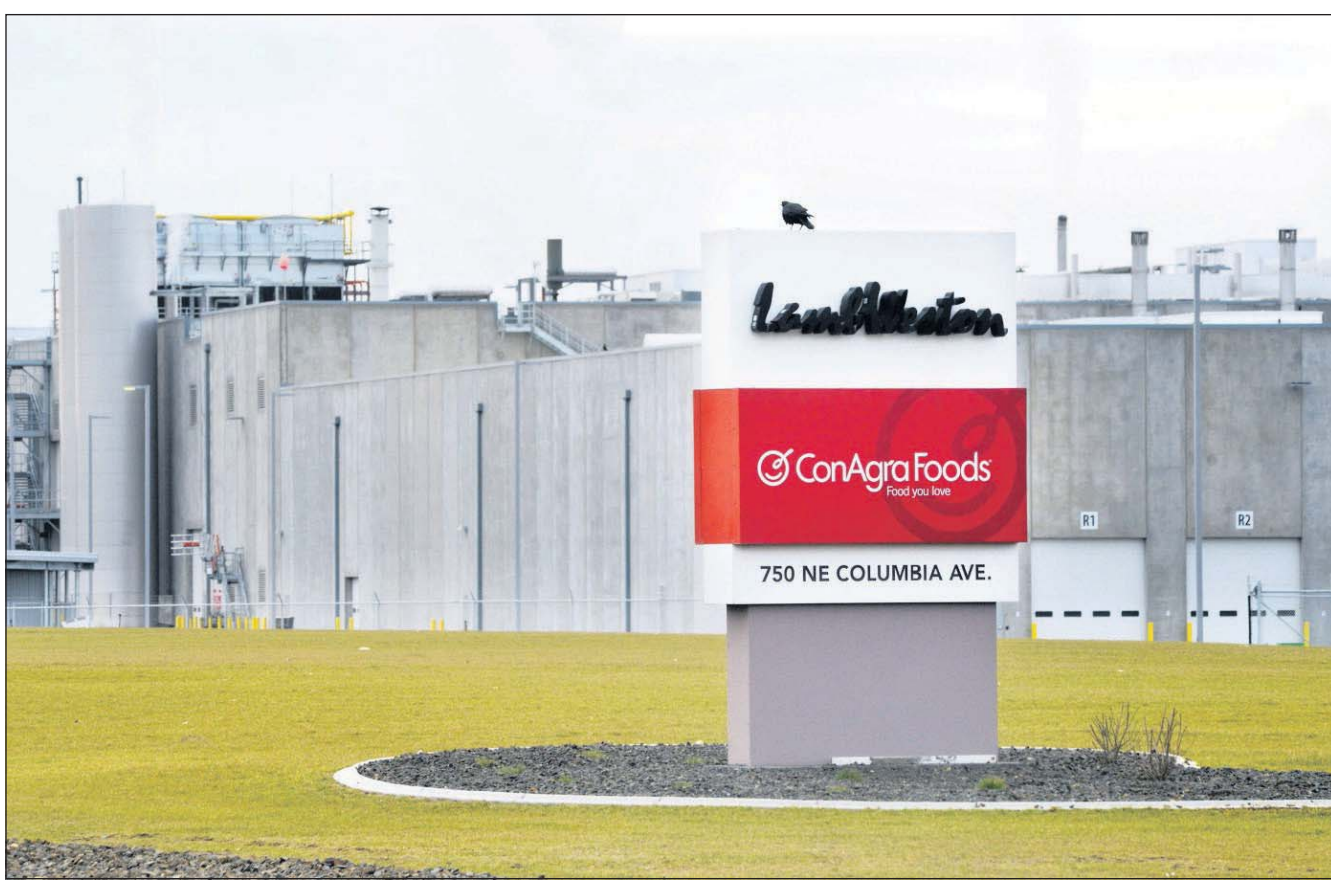
The Port of Morrow saw new investments in 2014 with the $200 million expansion of the Lamb Weston frozen potato facility.
