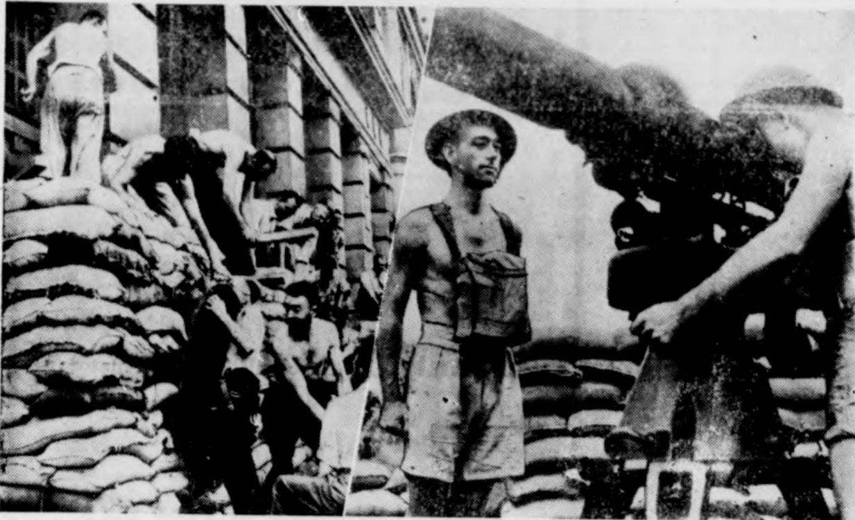
There is no city in Australia that can quietly sit back with the assurance that it will not be bombed by Japs. In the picture at the left, Melbourne city employees are doing their Australia-day task, erecting an ARP sandbag barricade outside of their working premises. Right: Members of the anti-aircraft battery man a height and range-finder at an action station in Darwin, Australia. The men work stripped to their waists.
