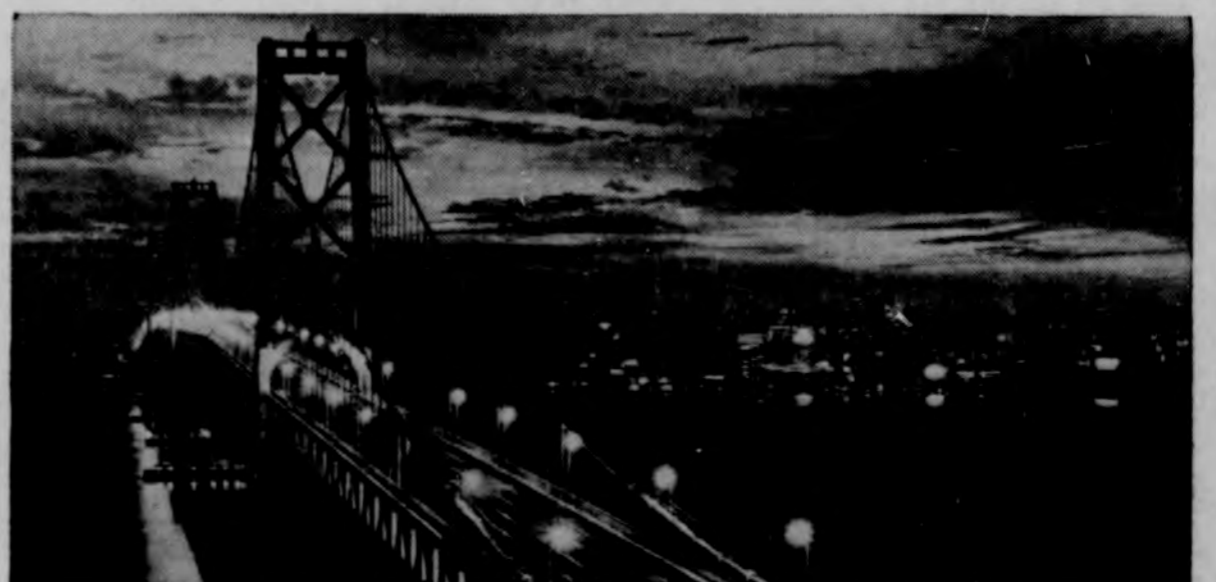
The world's largest sodium lighting installation, the first completed section of the Golden Gate bridge to Oakland, looking toward San Francisco from Yerba Buena island. Nine hundred and twenty-four sodium lights, the equivalent of 35 full moons makes the highway so bright that car headlights are unnecessary.
