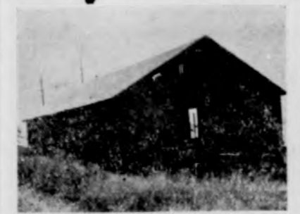
This picture is of the port building at Umatilla. It is on skids and is movable with the stage of river.
