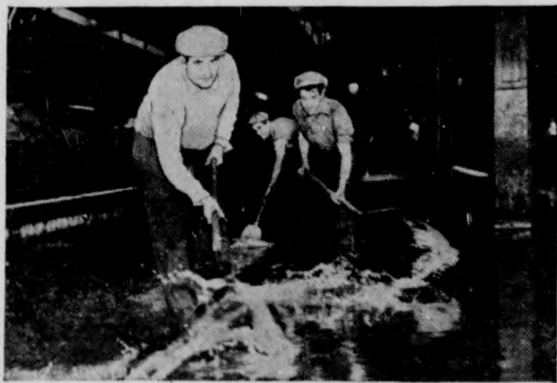
Photo shows workmen trying to clear tracks at the Union station in Chicago of a flood estimated at three to ten feet deep. A 36-inch water main burst putting 14 railroad tracks out of commission. The water also flooded portions of the new post office. Passengers from suburban trains were forced to alight from inbound trains about five blocks from the station. Damage was estimated at $200,000.
