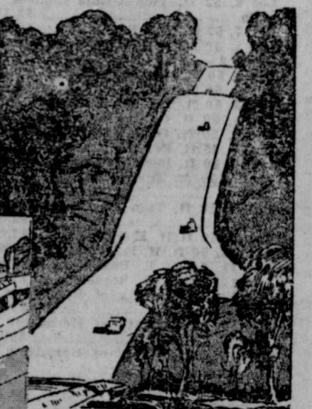
Very seldom are hills as steep as this. The average grade of highway hills is seven per cent. This hill is 25 per cent and a car must be good to make it.
