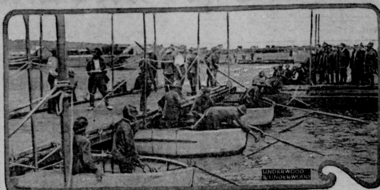
That the war of the Spanish against the Morocco tribesmen is "civilized," warfare is indicated by this photograph of Spanish engineers constructing a pontoon bridge in the fighting zone.
