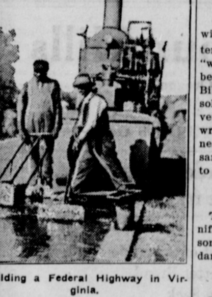
Building a Federal Highway in Virginia.
