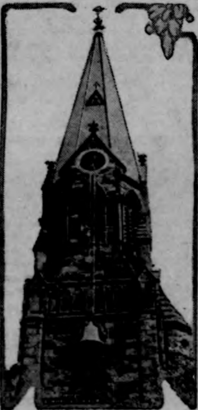
Installing bells in the tower of St. Mary's church, Washington, as a memorial to Rev. George Glatt. The bells are connected with a large Westminster clock so as to sound the hour in chimes. They vary from two to five feet in size.
