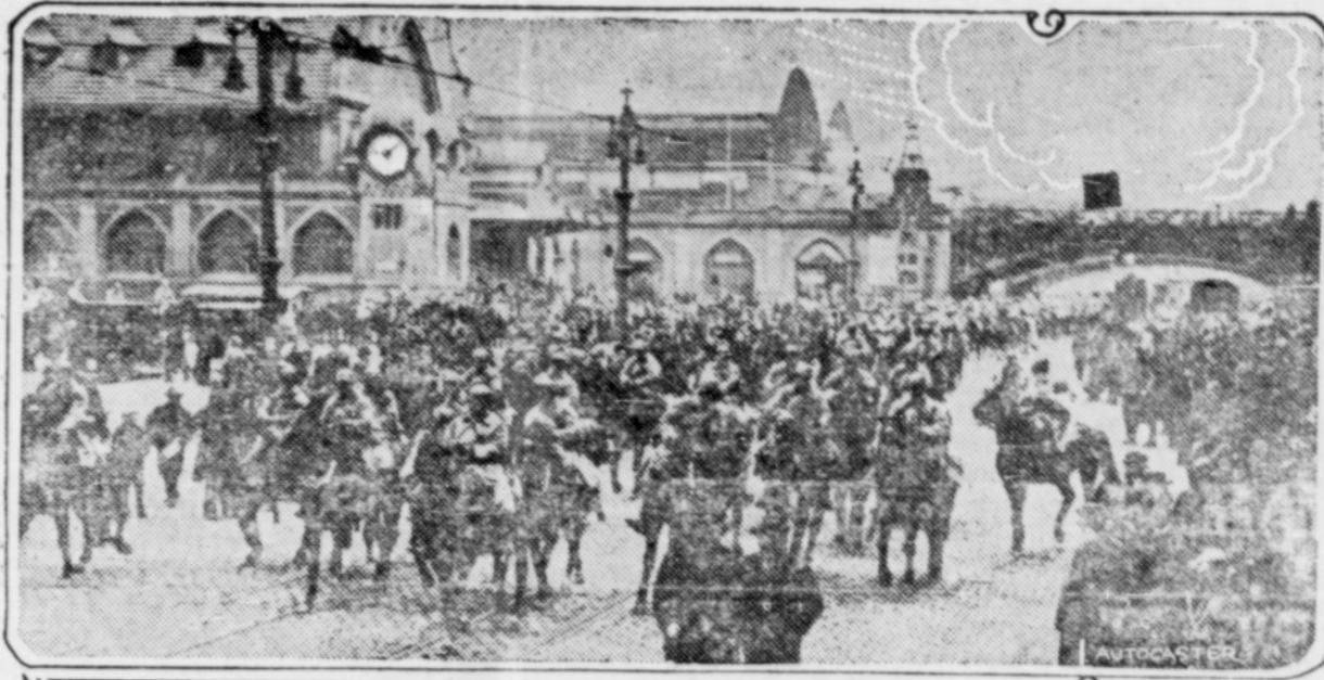
It was exactly 1.45 P. M. when the French cavalry rode into Essen, if the clock of the railroad station at left was correct. This exclusive picture is the first taken of the actual occupation of the German coal center by the French forces. Streets were crowded by Germans out to see the entrance of the invaders.
