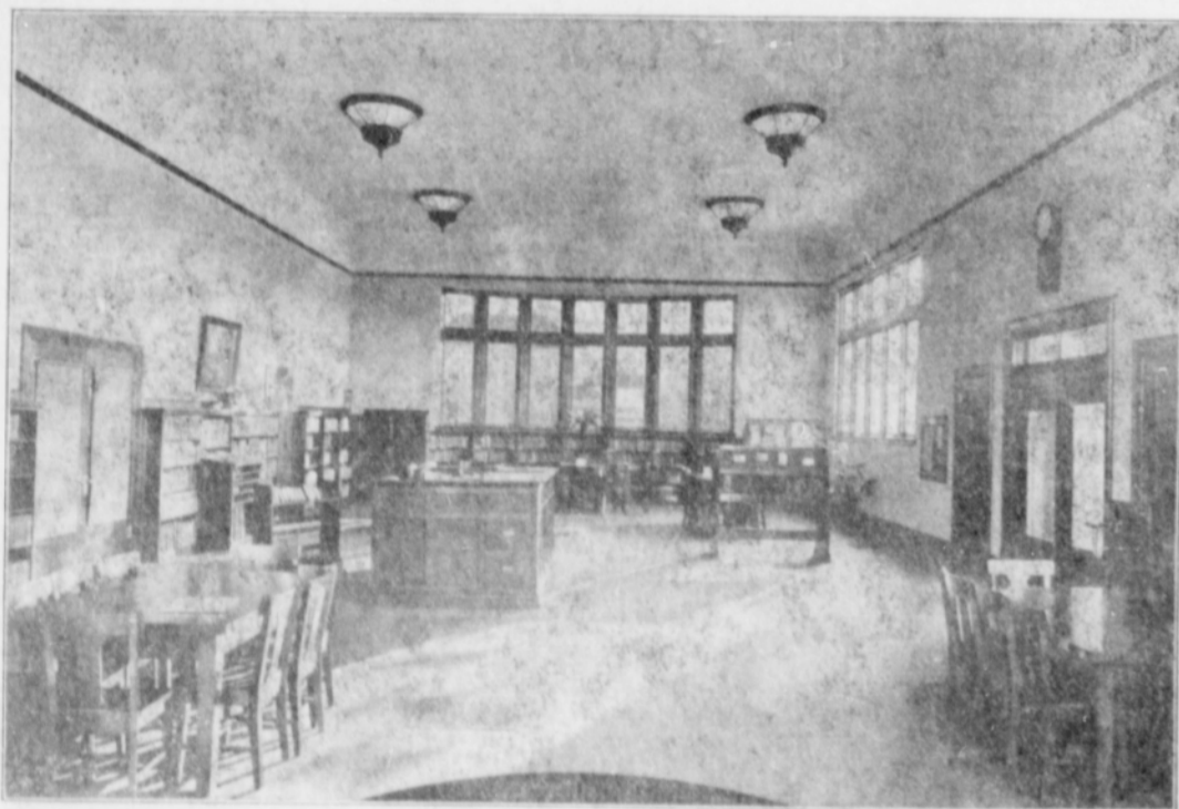
INTERIOR VIEW OF PORTION OF LIBRARY
