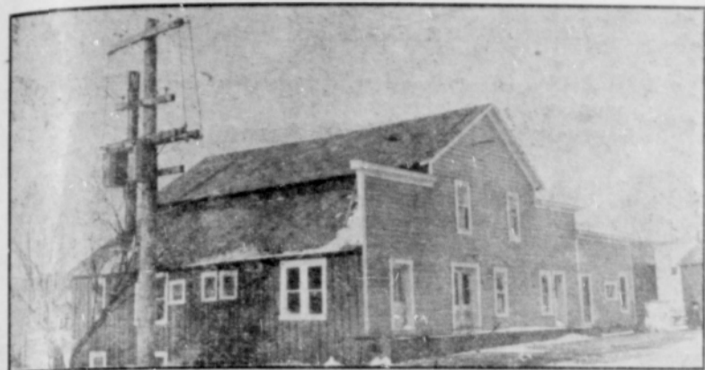
Old Cheese Factory Turned into a Starch and Dehydrating Plant.
