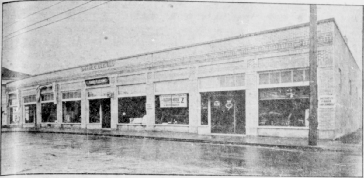
Typical of the progressive spirit of the town of Gresham is the new Ely building on Main street which was completed in October by D. C. Ely of St. Johns. Claude R. Stockton, a local contractor was in charge of the construction and the work was largely done by local men. Of attractive design and well located it is one of the most important additions of recent years. The building which is 80x100 feet is one story high.
