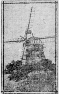
tion of the millstones the whole struc ture, including the machinery, is of wood. All the cog wheels are cut from native hard maple.
