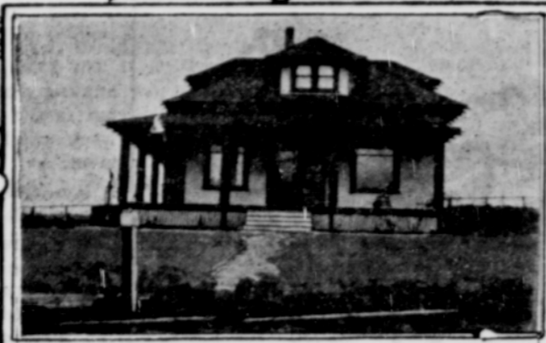
Recently built bungalow of Pat Collins on his fine farm on the south border of town. The place is well located with fine residences surrounding and is no longer "out in the country." The handsome new dwelling is the fruit of years of toil and saving and comes as a welcome blessing after many years of struggle.
