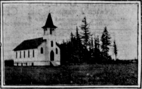
The latest addition to the devotional edifices of Gresham is the new Catholic church. It was conceived a year ago, erected during the past summer and dedicated early last fall. In charge of Rev. Father Bruenagel and sustained by a zealous congregation it rank is with the progressive places of worship and its worth is inestimable to the community.
