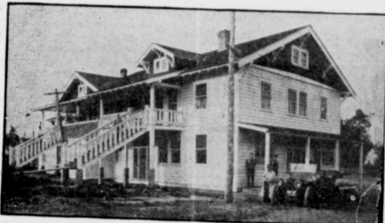
Upper Floor—Residence of J. W. Roots and Wm. A. Morand. Lower Floor—J. W. Roots & Co.'s Mercantile Establishment.
