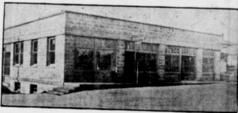
Wm. A. Morand's New Concrete Building, Containing Postoffice and Drug Store.
