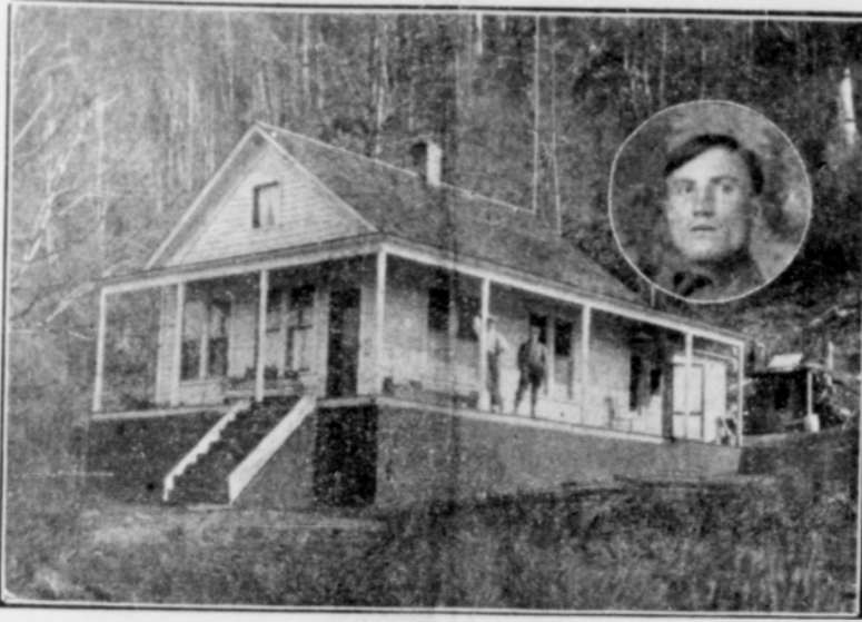
Farmhouse of Springhill Farm, Jenne Station; Walter Metzler, Manager
