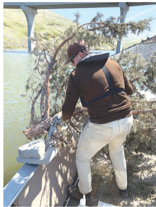
ODFW staff prepare to anchor a juniper tree to the bottom of Willow Creek Reservoir. -Contributed photo
