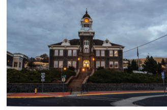
Morrow County Courthouse
