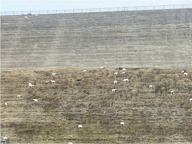
Petty’s goats eating the grass and weeds on the face of the spillway. - Photo by Chris Sykes
