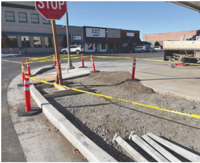
Sidewalk construction along Hwy 74 and Main. -Photo by Annalynn Black
