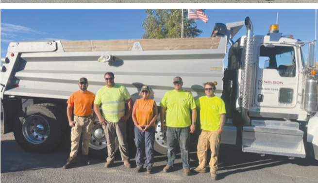
Silver Creek fills in hole with asphalt. -Photo by Leann Lankford
