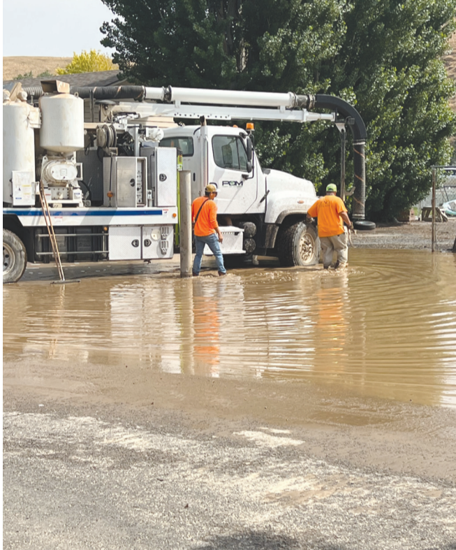
Port of Morrow employees work with a vacuum truck to get water off Ione's streets Monday. -Contributed photo
