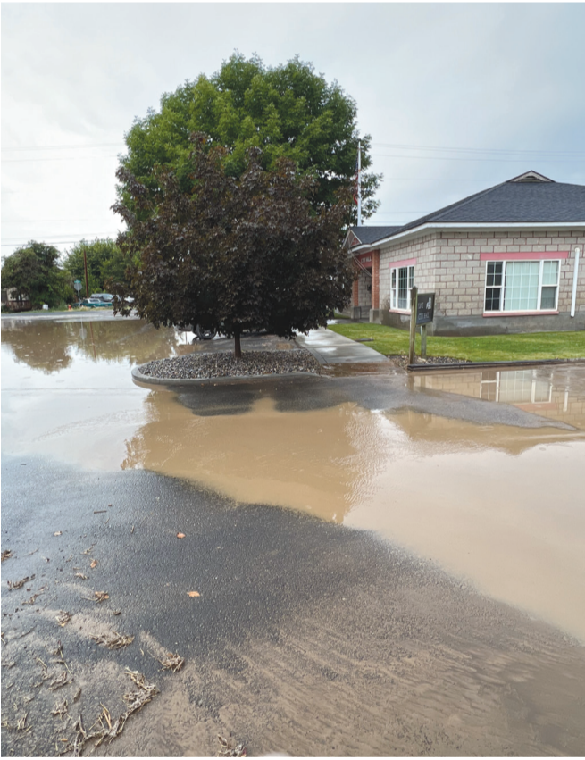
The water that covered Ione's 2nd Street also crept into Ione City Hall, causing city staff to relocate for the time being. -Contributed photo
