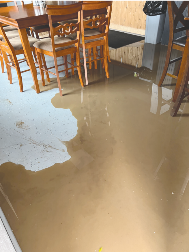
Flood water creeps across the dining area floor at Cardinal Café in Ione. -Contributed photo
