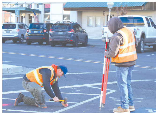
Surveyors work on Main Street in Heppner as part of a larger ODOT project that includes altering sidewalk wheelchair ramps. -Photo by Andrea Di Salvo
