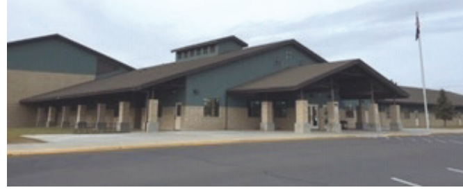
Windy River Elementary School in Boardman will be getting a new roof thanks to funding from Amazon, the Morrow County School District board of directors decided last week. -Contributed photo
