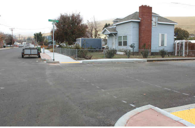
The City of Heppner is still awaiting contractors to put the finishing touches on several Heppner streets, but city workers are putting in time to make sure safety requirements are met. -Photo by Andrea Di Salvo
