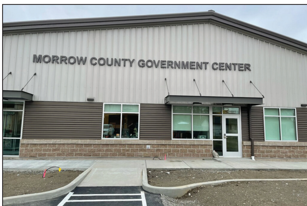
The new county office buildings have been completed and are now open for businesses in Irrigon
